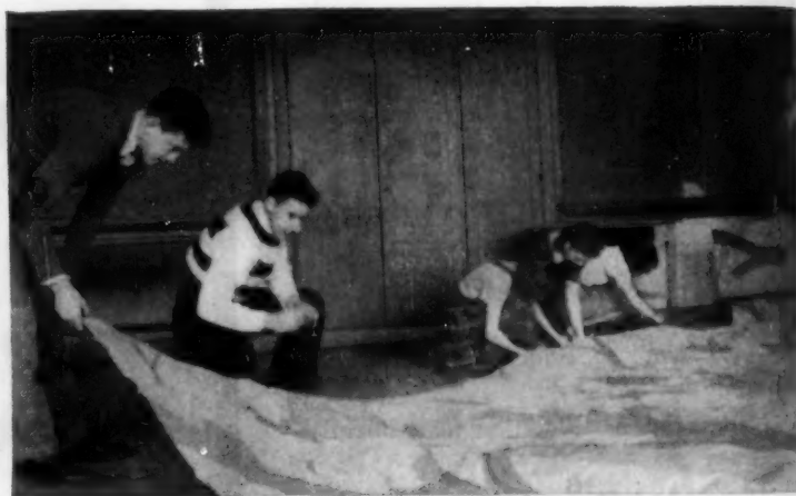
Inserting the bent wire hangers
