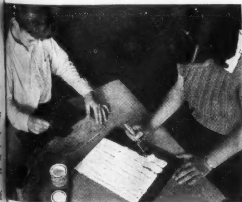
7—Applying shellac and crackle lacquer
