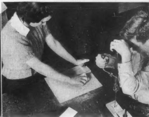
6—Sanding surface, boring holes for laces
