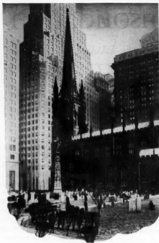
Down in Trinity Churchyard, at the head of Wall Street's canyon
