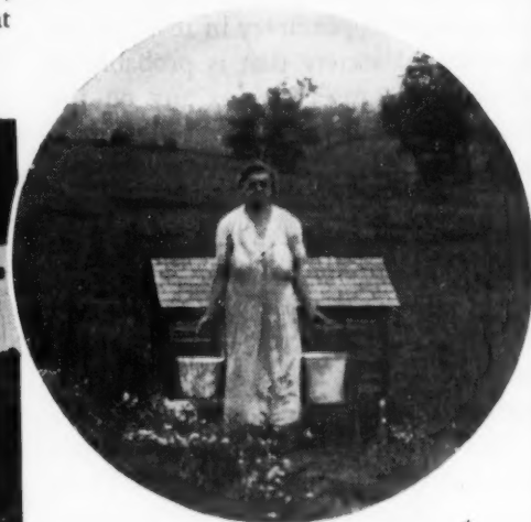
Electricity—which is being made available to rural America thru the Rural Electrification Administration—lightens burdens
