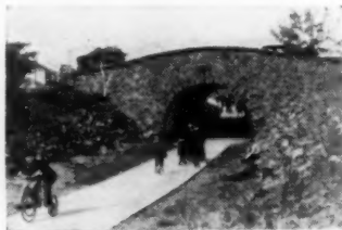
Courtesy, City Housing Corp. Pedestrian underpass, Radburn, New Jersey
