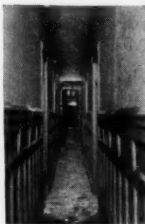
Courtesy, Building America
