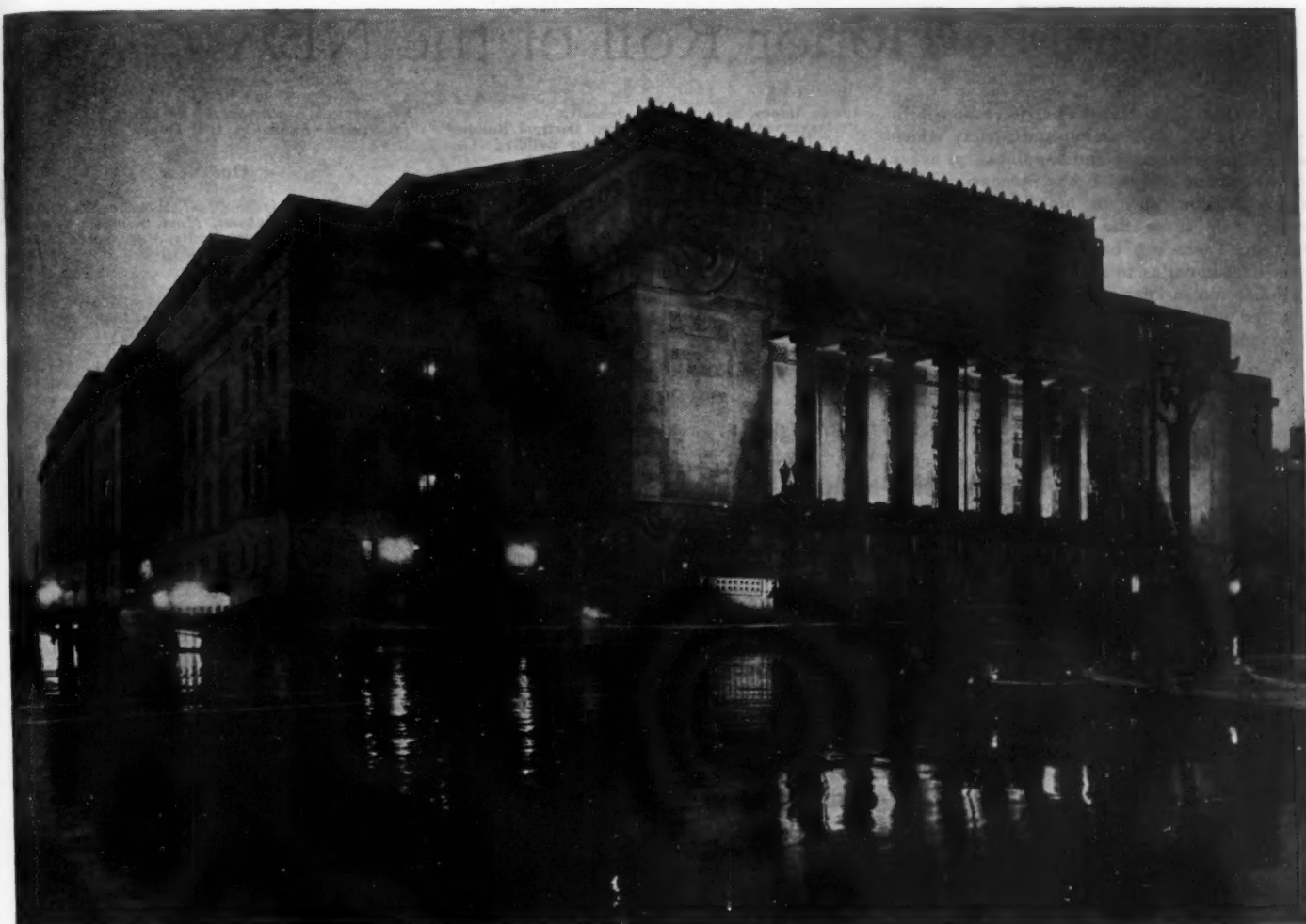
The beautiful new St. Louis Municipal Auditorium where the Department of Superintendence will meet the last week of February
