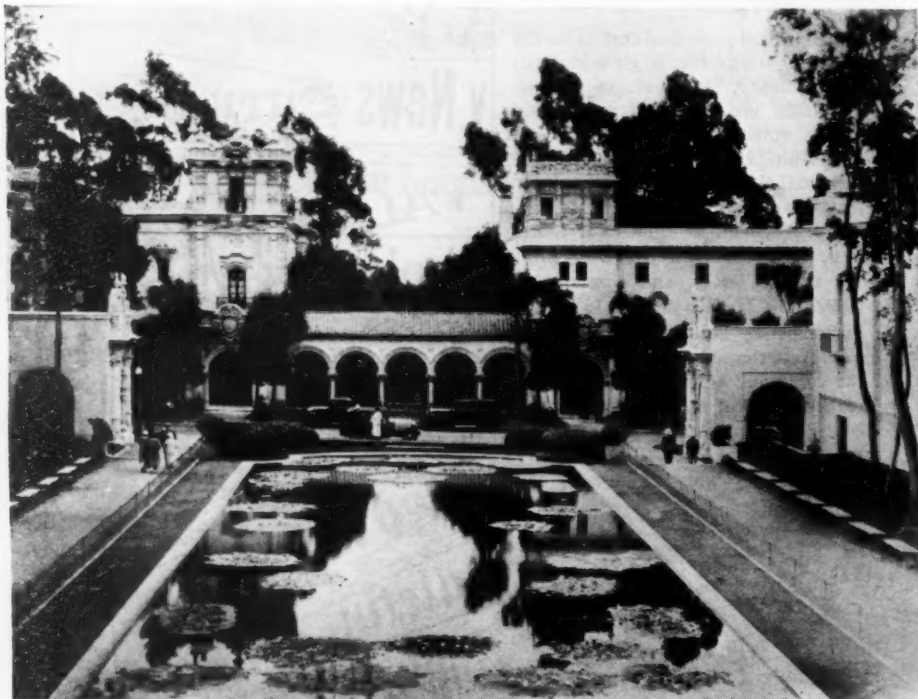
Palace of the Modern Home; House of Hospitality
