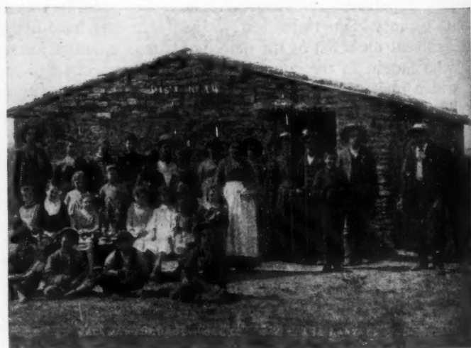
ON THE LEFT: Sod-house home. On the right: Sod schoolhouse of the Kansas frontier. These were built by laying blocks of sod on top of each other and on top of the roof. Such houses were warm in winter and cool in summer.
