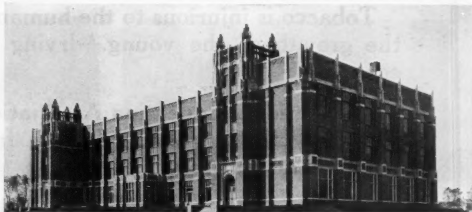
Mt. Vernon Elementary School, Chicago, Illinois
