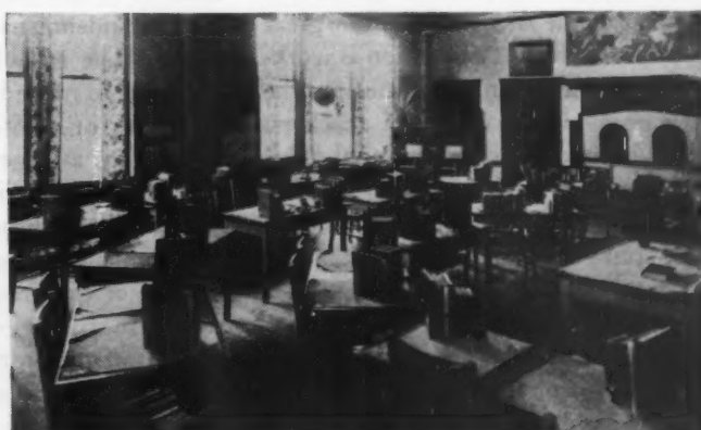
Even the upper grade rooms of the modernized school have a flexible environment suitable for active work. This sixth grade classroom of the training school of Milwaukee State Teachers College is an example.
