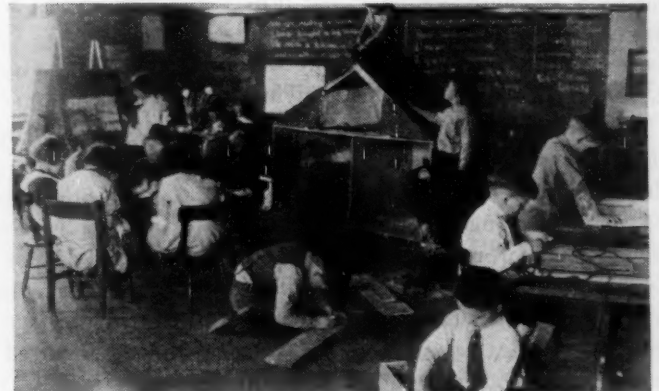
A box house is here seen in the process of construction, and furniture, rugs, and curtains are being made for it. These children of a Kalamazoo public school are learning lessons which they will always remember.
