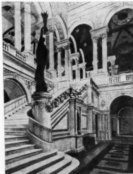
THIS STAIRWAY in the entrance hall of the Library of Congress has been styled "a vision in polished stone." The noble building of which it is a part is a tribute to the heritage of the ages recorded in books.
