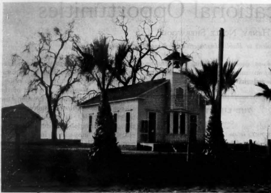
THE SLOUGH SCHOOL in Sutter County, California, is typical of many country schools in the northern part of the state. Without the palm trees, there would be nothing to distinguish it from rural schools in other states.
