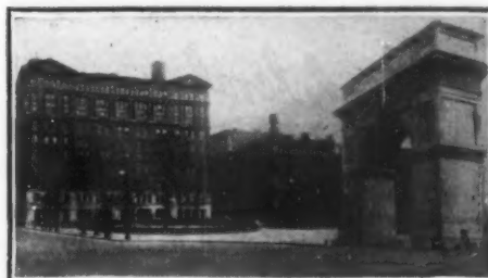
University Buildings at Washington Square
