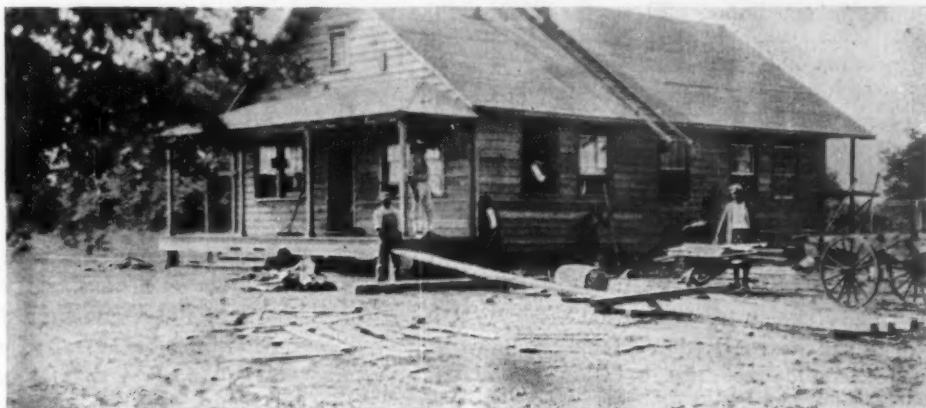
BOYS of the Penn Normal Industrial and Agricultural School at work on house demonstrated by Better Homes Committee, St. Helena Island, South Carolina, 1924.
