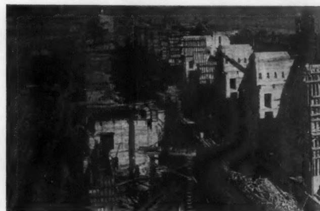
Construction work at Muscle Shoals
