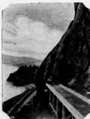
APPROACH TO TUNNEL
