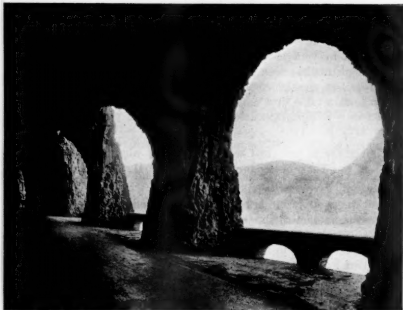
The Mitchell Point Tunnel hewn out of solid rock— part of the Columbia River Highway
