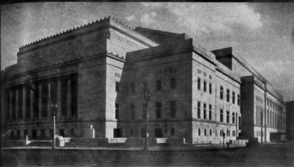
The Municipal Auditorium and Community Center Building, where our meetings are to be held
